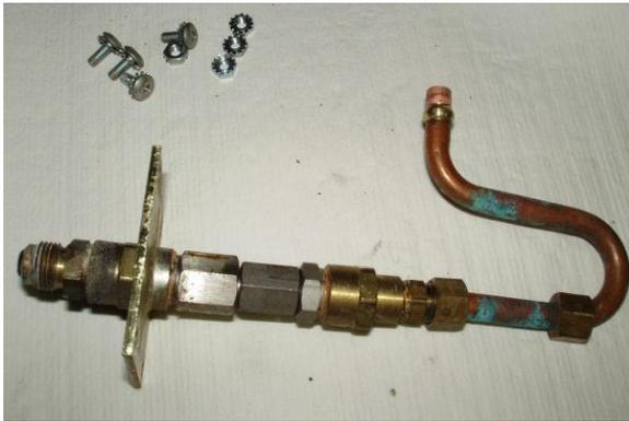
3. Remove the 4 x Nuts/Bolts securing the bulkhead fitting (a second pair of hands is recommended to do this)
