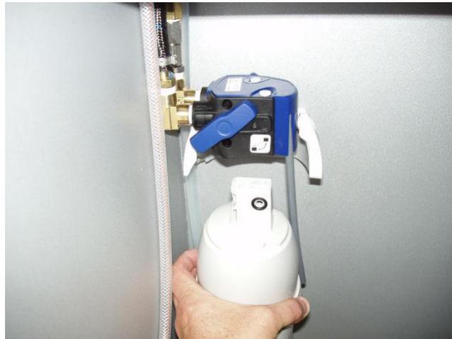
11) Ensuring the locking handles are in the FULLY UNLOCKED position as shown and install the filter cartridge
