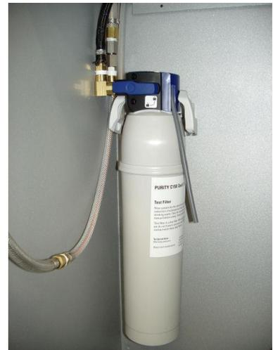
13) Re-connect the power cord and turn ON the water supply to refill & reheat the heater tank and also check for leaks
