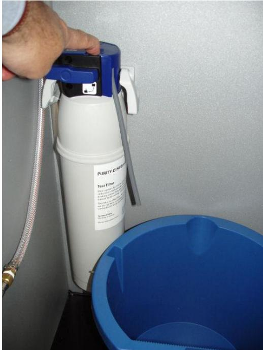
13) Operate the spray hose (not shown) for 20 seconds to drain-off some water from the heater tank, whilst the tank is refilling press the 'purge' button on the top of the filter head to purge out any air or carbon dust from the cartridge
