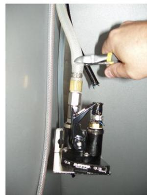
3) Select either of the 2 x #10-24 or #10-32 x 1" screws in the kit and introduce to the same threaded inserts that the original screws were removed from, screw-in a few turns only using fingers
