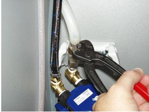
9) Push both sections of tubing onto the barbed fittings and pinch the hose clamps to seal/secure
