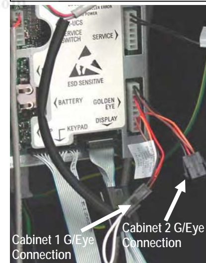
Photo 2 – Á LA CARTE Golden Eye connection in a 311 Tower using Cabinet 1
